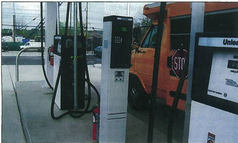
A school bus at a fueling site equipped with Gilbarco's Gasboy system
